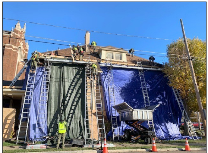
Pictures of Groover Roofing & Siding replacing the rectory roof.
